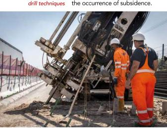
The purpose of the consolidation works is to improve the physicalmechanical characteristics of the soil behind the excavation section - behind the piers and the cap – for a thickness of about 3m.
